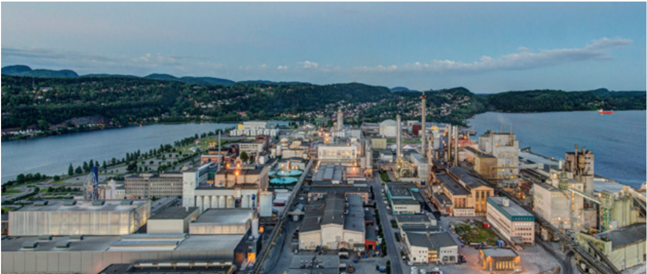
Herøya Industripark will test new groundbreaking climate technology. Photo: Herøya Industripark.
